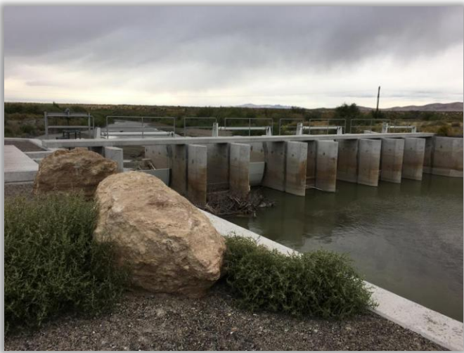
Pitt-Taylor diversion works on the Humboldt River; delivers decreed irrigation to producers such as the Flying M Ranch.
