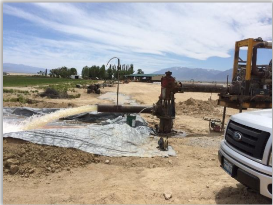
2014 Pump testing a new irrigation well in Big Smoky Valley (McLeod Ranch)
